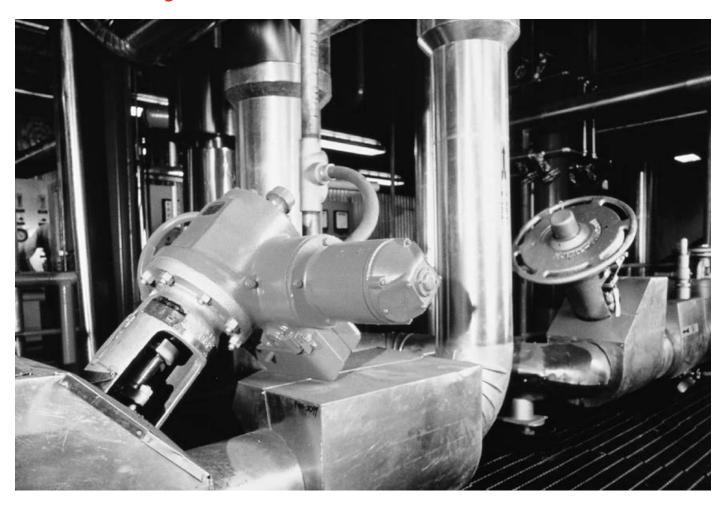
Flowserve Edward Valves supplies actuators for Edward forged and cast steel valves when alternate sources of power are required to open, close or maintain an intermediate position in the valve.
