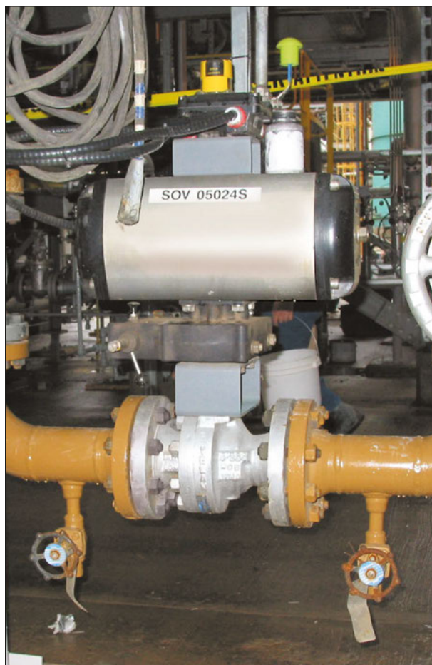
Automated split-body ball valve on hydrocarbon service at a Petro Canada refinery in Montreal, Quebec. The valve has been cycling every hour 24/7.
