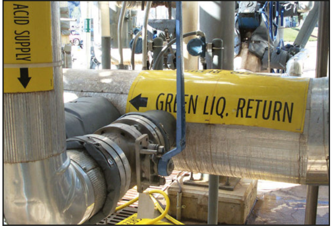
Split-body ball valve in pulp and paper.
