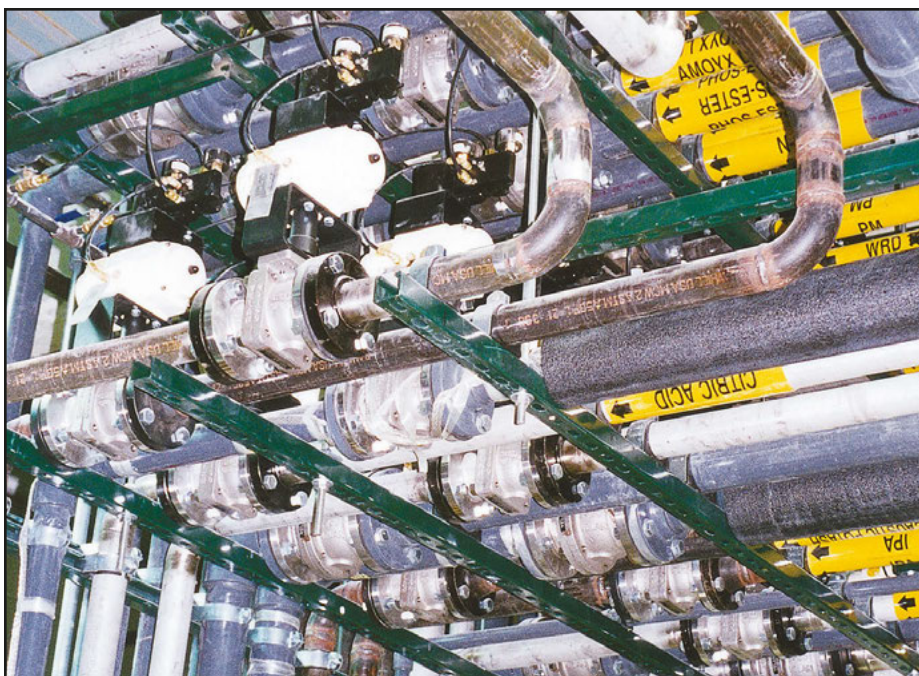
Velan split-body automated ball valves sizes NPS ½ – 4 (DN 15–100) installed in a major chemical plant, in Ohio.
