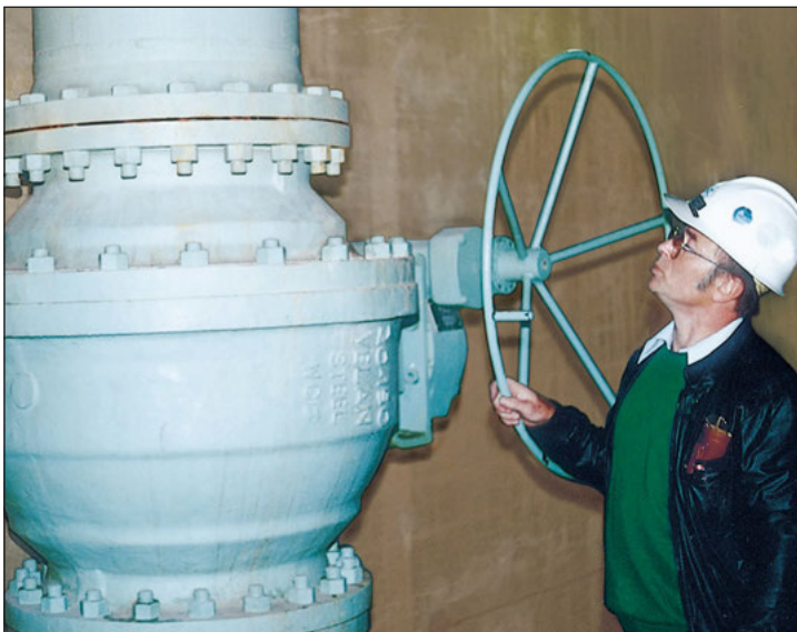
NPS 20 (DN 500) split-body bypass ball valve installed at James Bay in Canada.
