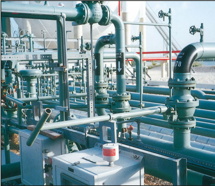
Installation of NPS 6 (DN 150) SB-150 with extension handle at a Texas refinery.
